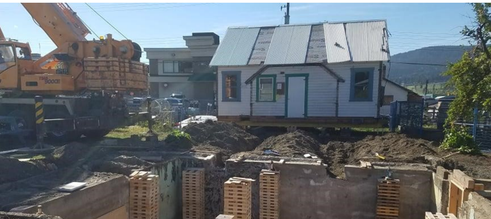
MOVING THE HOUSE OFF ITS FOUNDATION. PHOTO: OLIVER BERGER.
