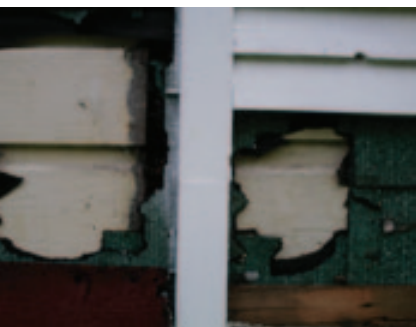
[Top] Uncovering the original siding
