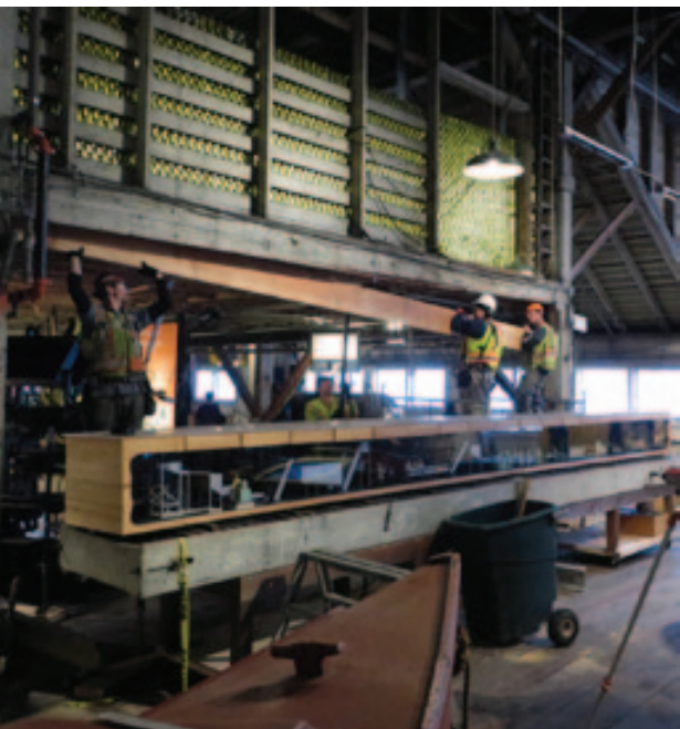
The Seismic 2000 construction crew setting a new lintel. Photo credit: Heidi Rampfl.
