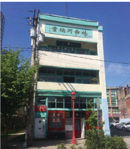
The 1903 Chinese Empire Reform Association Headquarters building.
